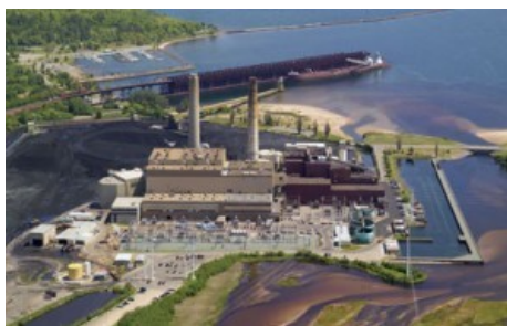
Presque Isle power plant Source: We Energies
